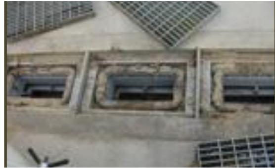
**Step 1.** Remove grates to gain access to filter/hydrocarbon boom. **Take photos** throughout maintenance procedure.
