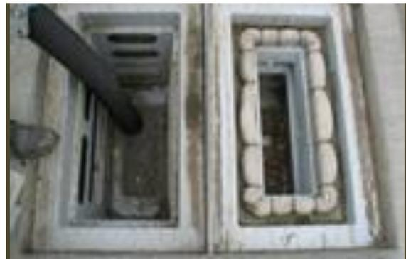
**Step 2.** Remove skimmer tray, vacuum out debris, and dispose in trash.
