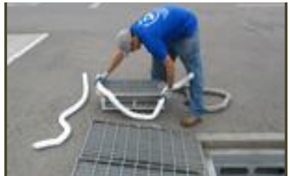
**Step 3.** Remove old hydrocarbon boom and replace with a new boom.
