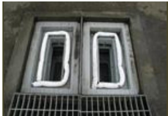
**Step 4.** Replace skimmer tray inside filter and replace grates over the filters.
